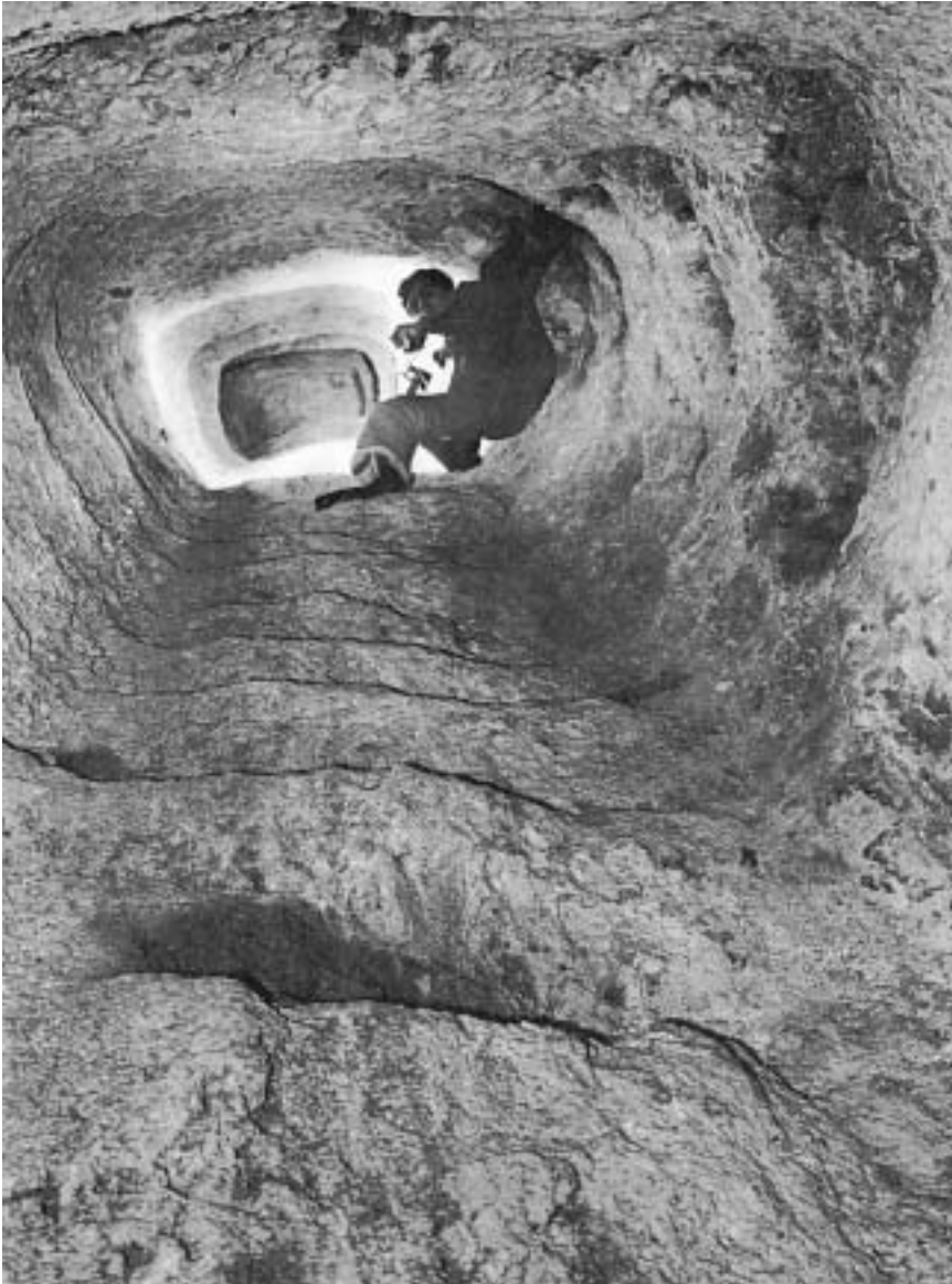
A Ventilation Shaft of the Tunnel in the Ein-Aroub Aqueduct (photograph: Ami Erev).
