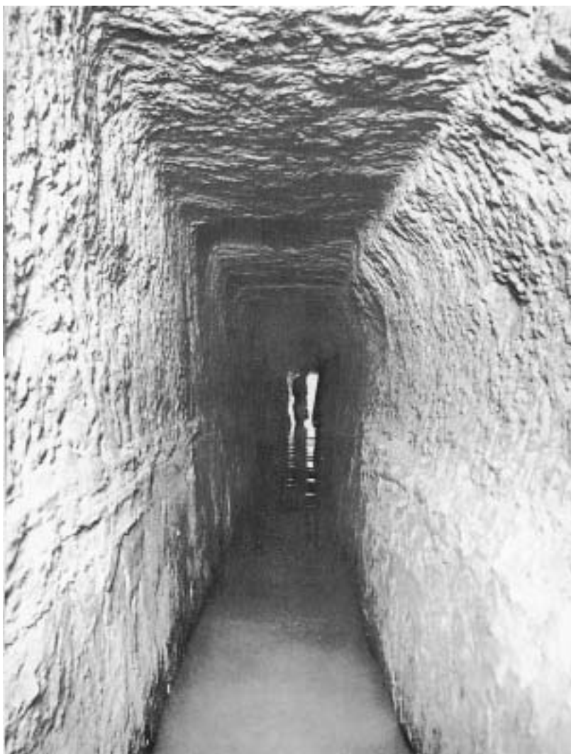
The Shiloah Tunnel in Jerusalem (photograph: Ami Erev).
