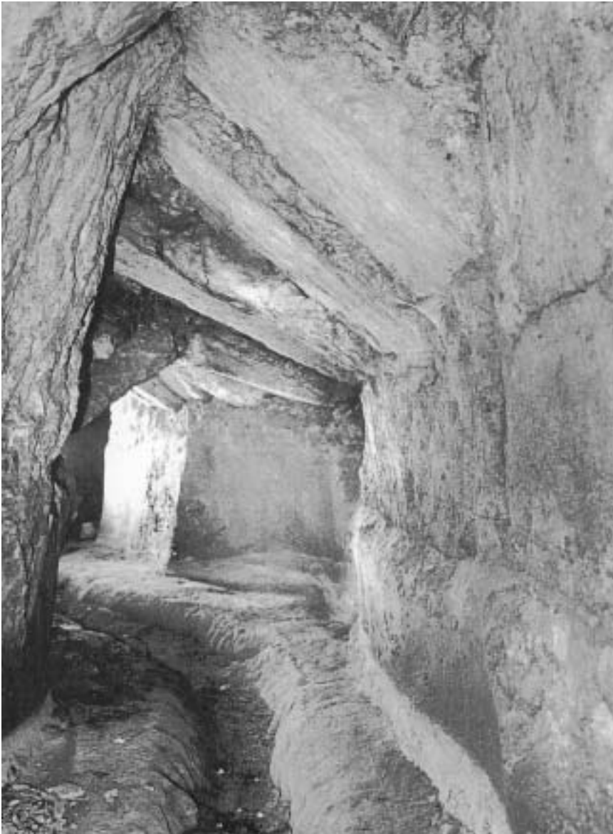
A Tunnel in the Ein-Aroub-Jerusalem Aqueduct (photograph: Ami Erev).
